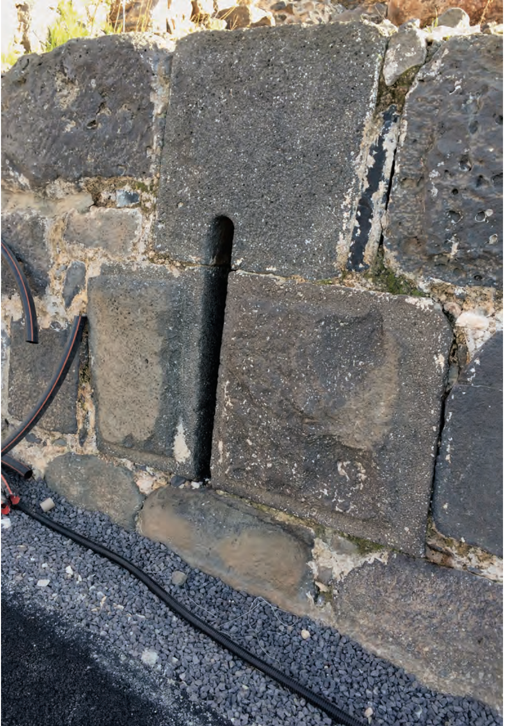
Belvoir, exterior of one of the embrasures of the inner enclosure. ( Michael Fulton )
